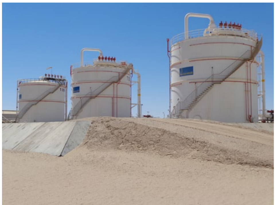
□ Wintershall oil storage tanks, Libya
