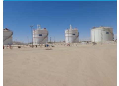
□ Wintershall oil storage tanks, Libya
